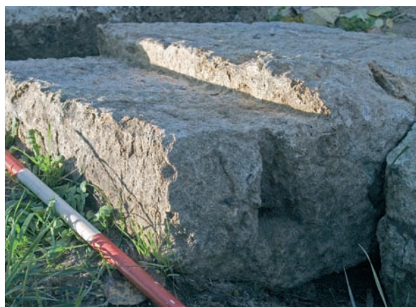
Fig. 12. Carved blocks with holes for clamps
