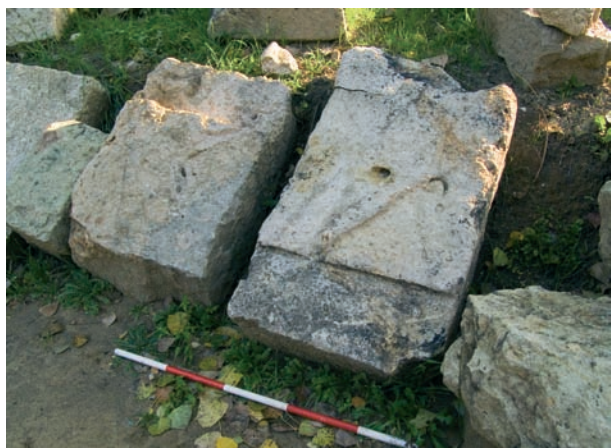
Fig. 11. Carved blocks with holes for clamps
